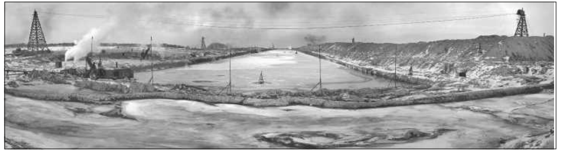
EXCAVATION of the Livingstone Channel in the Detroit River, 1910.
