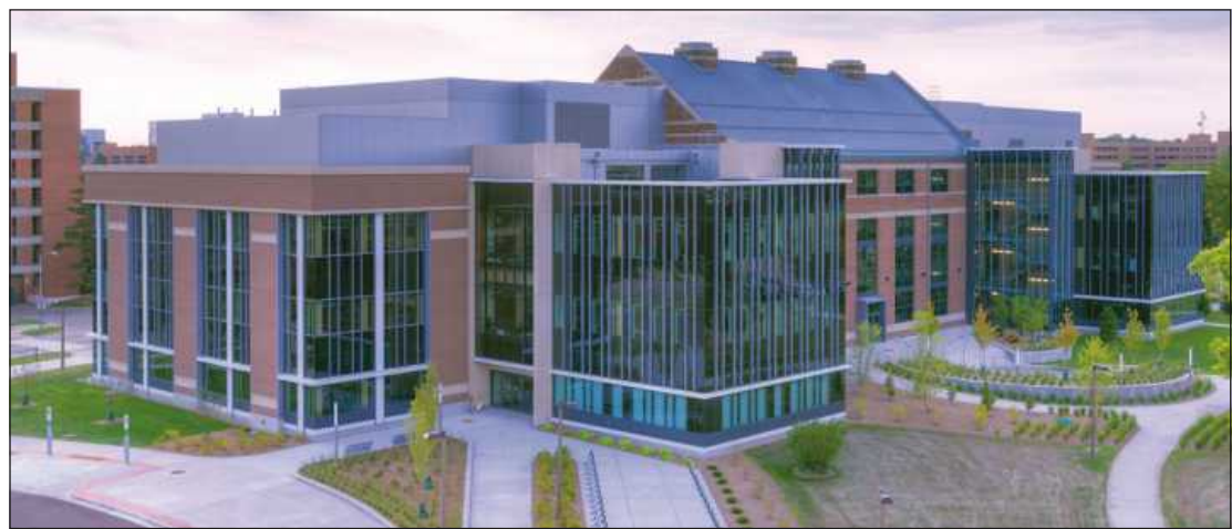
THE SHAW LANE power plant on the Michigan State University campus in East Lansing was in service from 1947 to 1975. Over the past few years, Granger Construction and its building trades union workforce converted the building, built additions, and created classroom and laboratory space. Over the past several months the building's design has won two awards for its creative use of mass timber.
